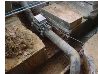
**CALIPER** - Geometric Inspection
